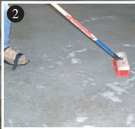
2 Scrub floor with degreaser
