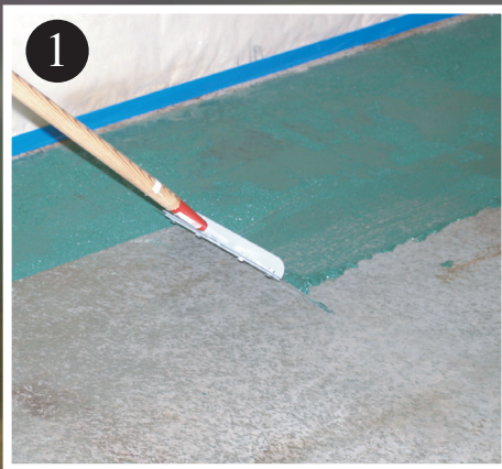
1 Scraping softened epoxy floor paint
